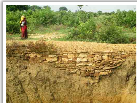
Reinforcement of the edges of Ram Balak's pond
