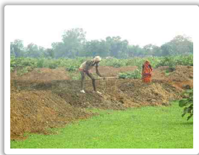
Construction of small dikes retaining rainwater on cultivated land
