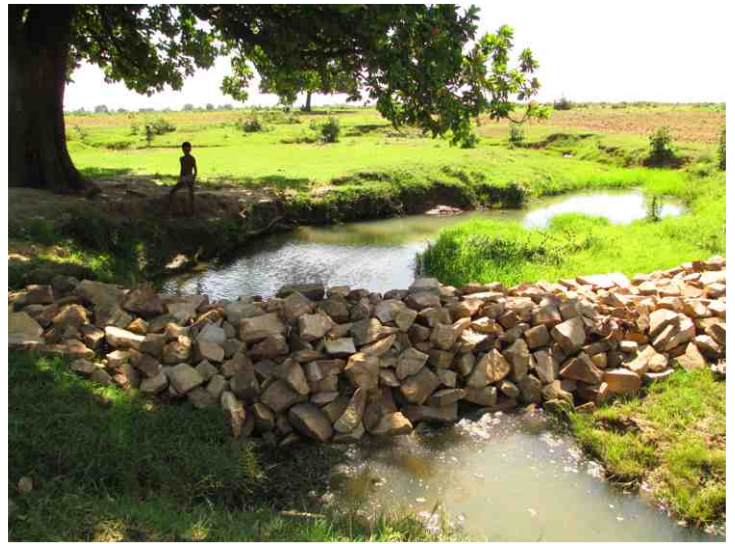
Stone check dam to slow water flow and help it infiltrate the soil
